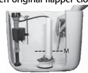
c) Flush & hold to drain water. Place bucket. Disconnect water supply line.
