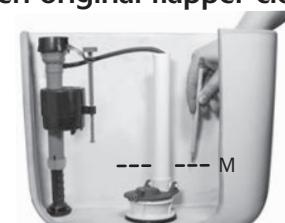
c) Flush & hold to drain water. Place bucket. Disconnect water supply line.
